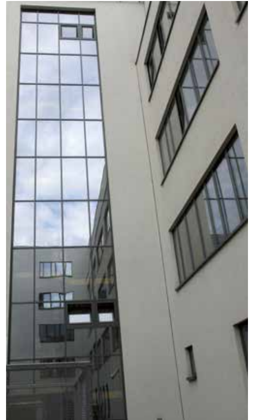
HOSPITAL KLADNO, PART A Investment excluding VAT 599 million CZK Reconstruction of the hospital monoblock.
